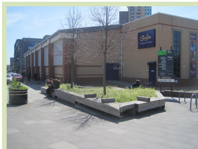
Existing planters requiring maintenance
